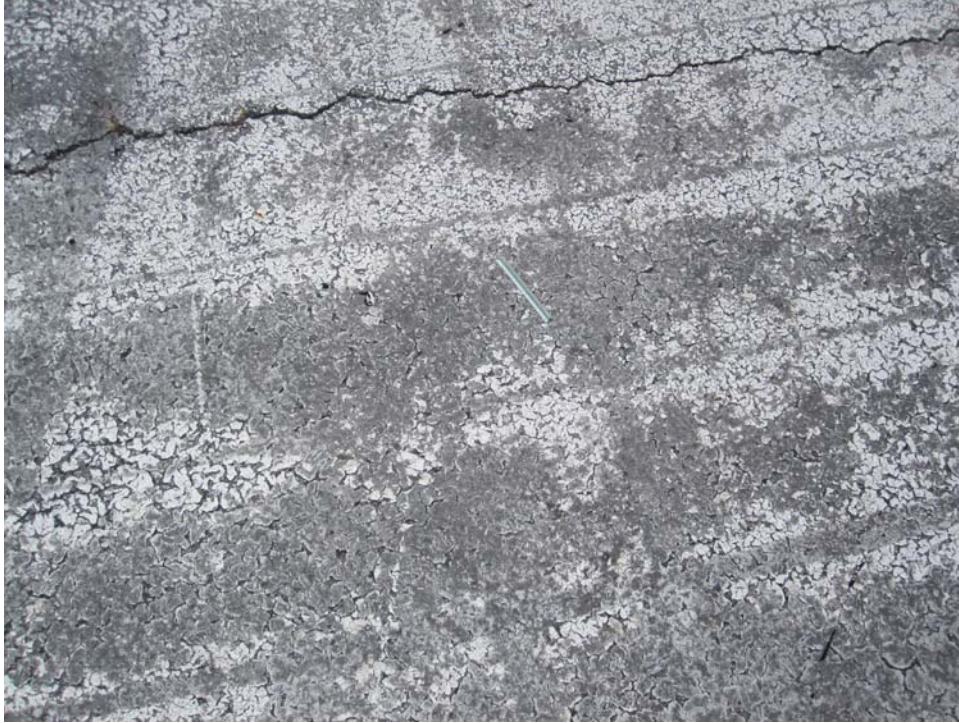
R1432AB-10. Unsatisfactory Paint (1).
