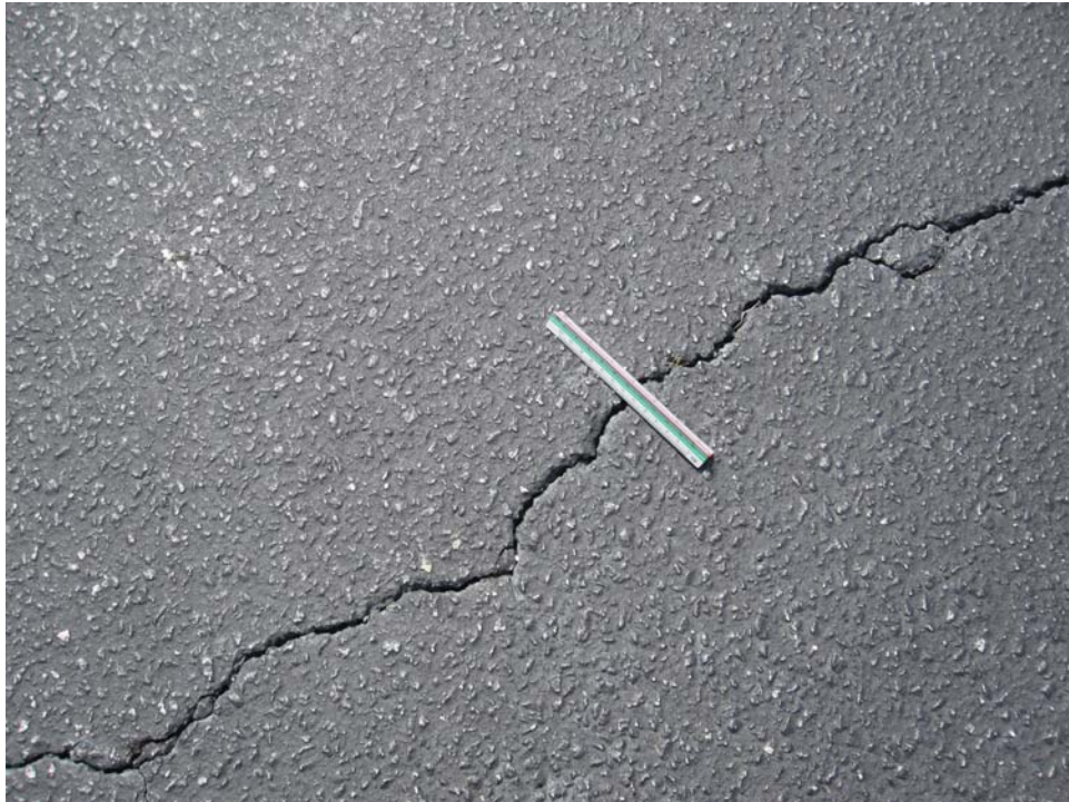
A01AB-10. Longitudinal and Transverse Cracking (Sample Unit #04).
