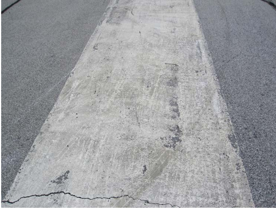
R927AB-10. Unsatisfactory Paint.
